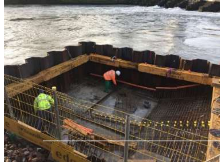
Figure 7: The coffer dam is constructed
