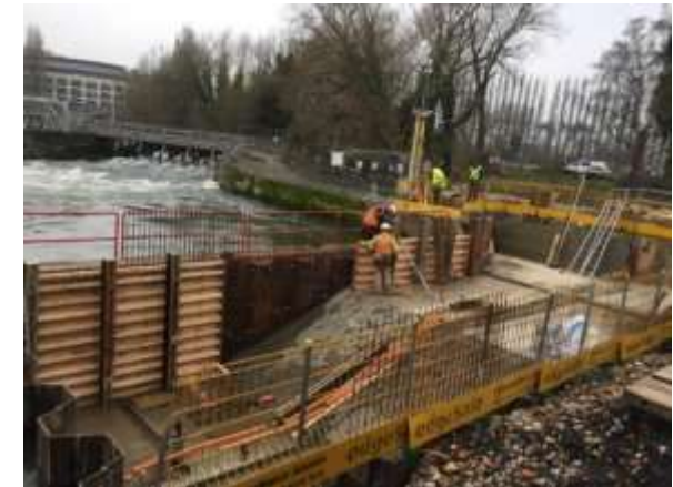
Figure 8: The concrete formwork begins to take shape
