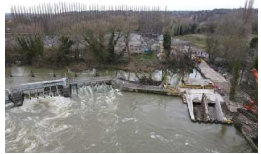
Figure 1: Site in February 2021, showing civils work abutting embankment
