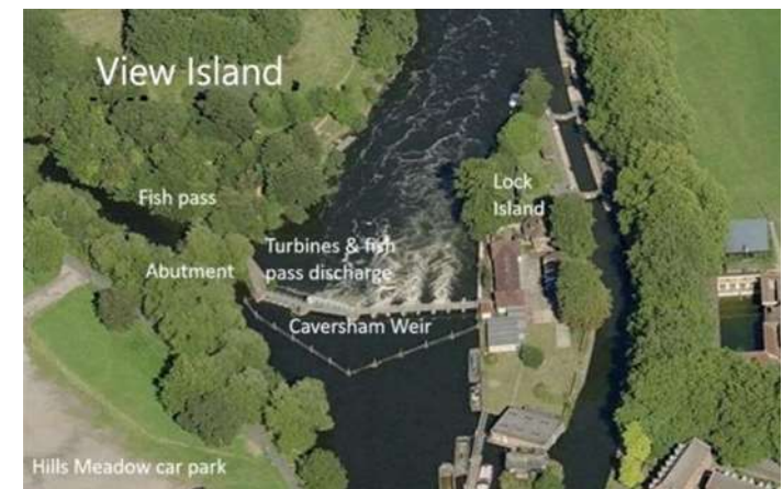
Figure 3: Aerial view of the site at Caversham Weir showing the location of the fish pass and turbines
