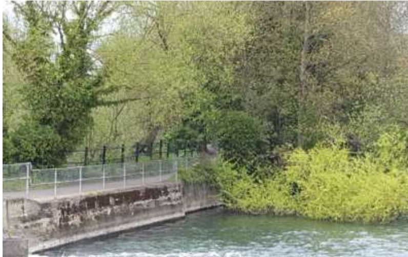
Figure 2: Part of the embankment showing the footpath before work started
