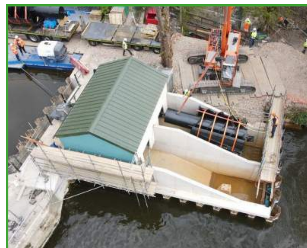
The turbines being installed
